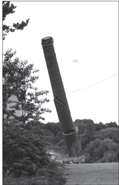
The Elliot and Son's greenhouse chimney was demolished on July 7, 2016. J. Davis
